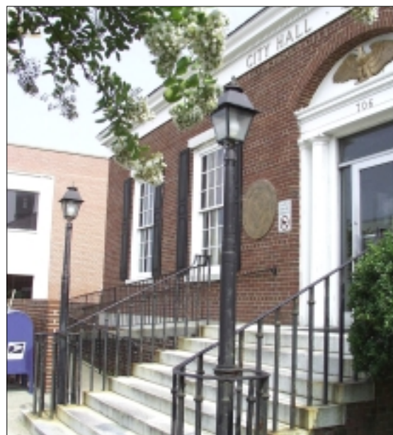
A ramp located next to the stairs to this town hall provides an accessible entrance.
