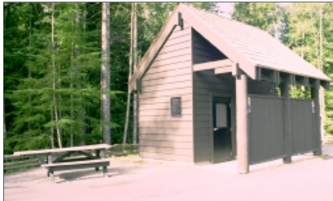
Public toilets at a park were built to comply with the new construction requirements of the ADA Standards.
