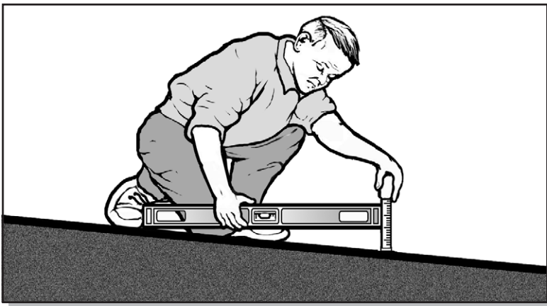
Measuring slope using a 24-inch level and tape measure
